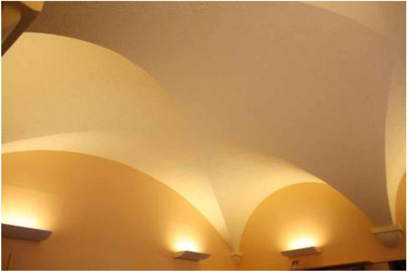
Vaulting and corbels to ceiling – ground floor east wing
