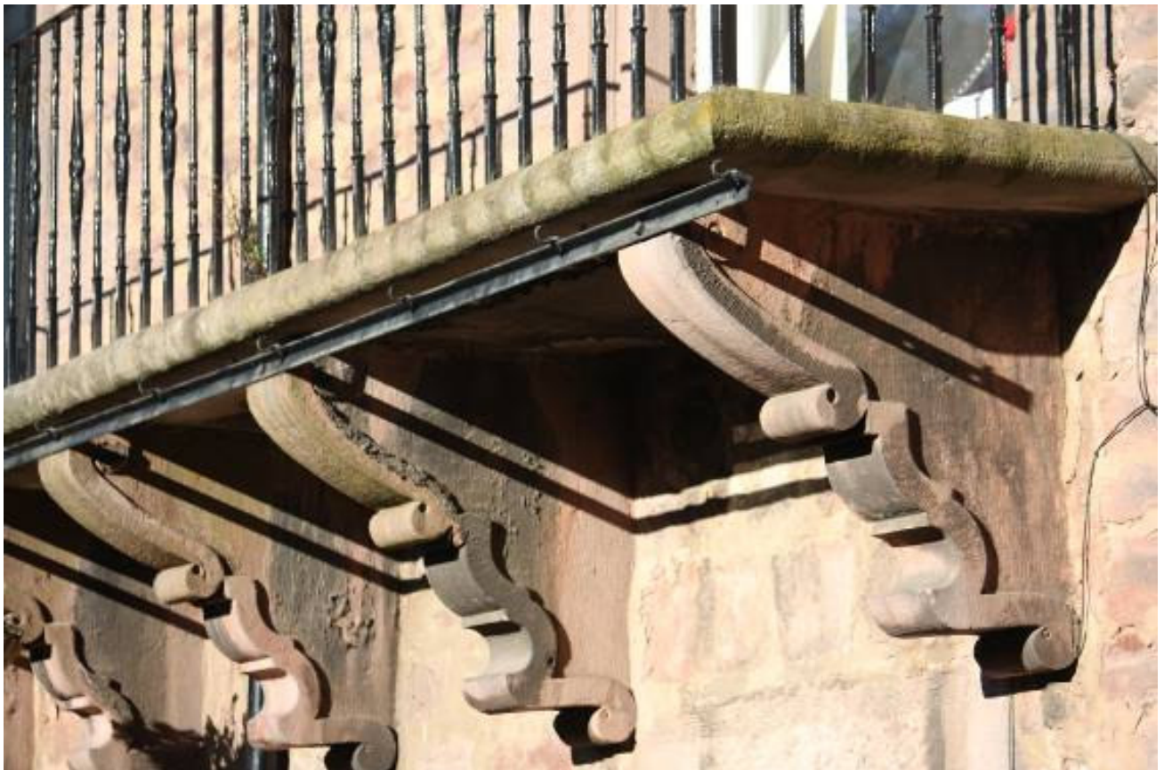
Environmental staining to balcony and evidence of plant growth
