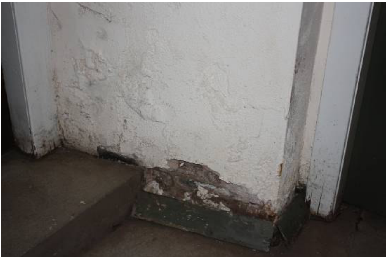
Evidence of damp internally at ground floor
