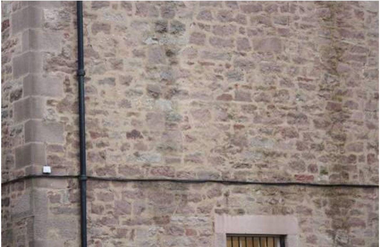
Staining to north elevation due to damaged rainwater goods
