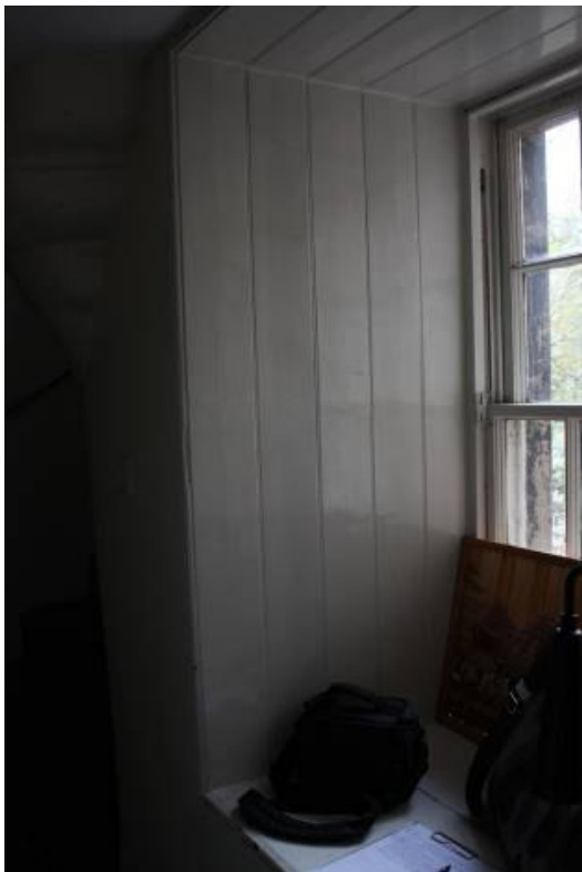
Example of window with mix of tongue & groove and raised and fielded panelling
