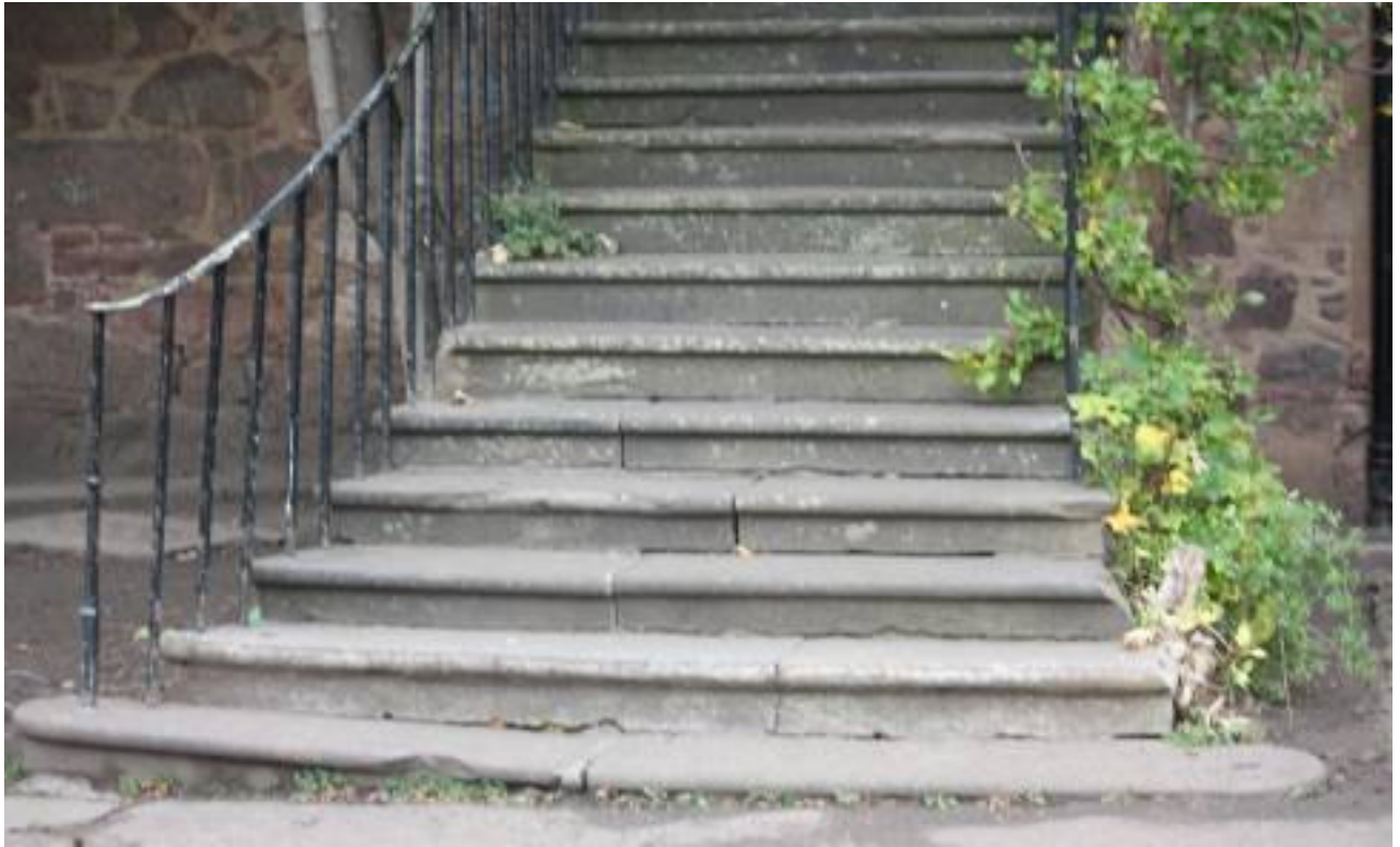
Staircase to Head Teacher's office showing damage to stone structure, steps and balustrades.
