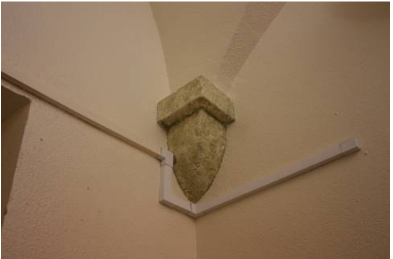
Vaulting and corbels to ceiling – ground floor east wing
