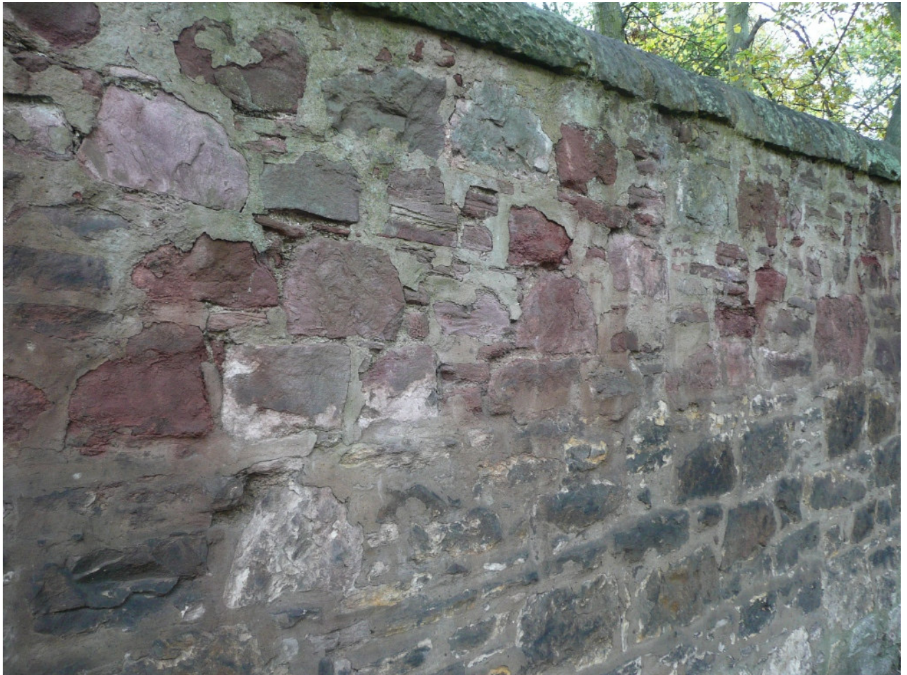
Damage to stonework and copes on north boundary wall
