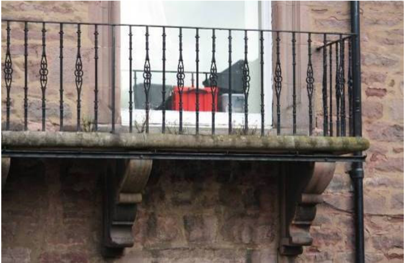
Environmental staining to balcony and evidence of plant growth
