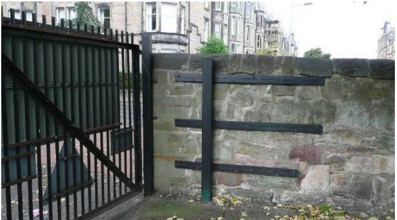
Metal straps to strengthen wall
