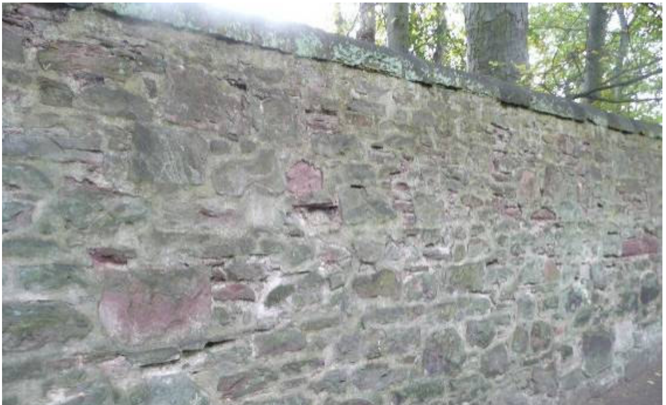
Damage to stonework and copes on north boundary wall
