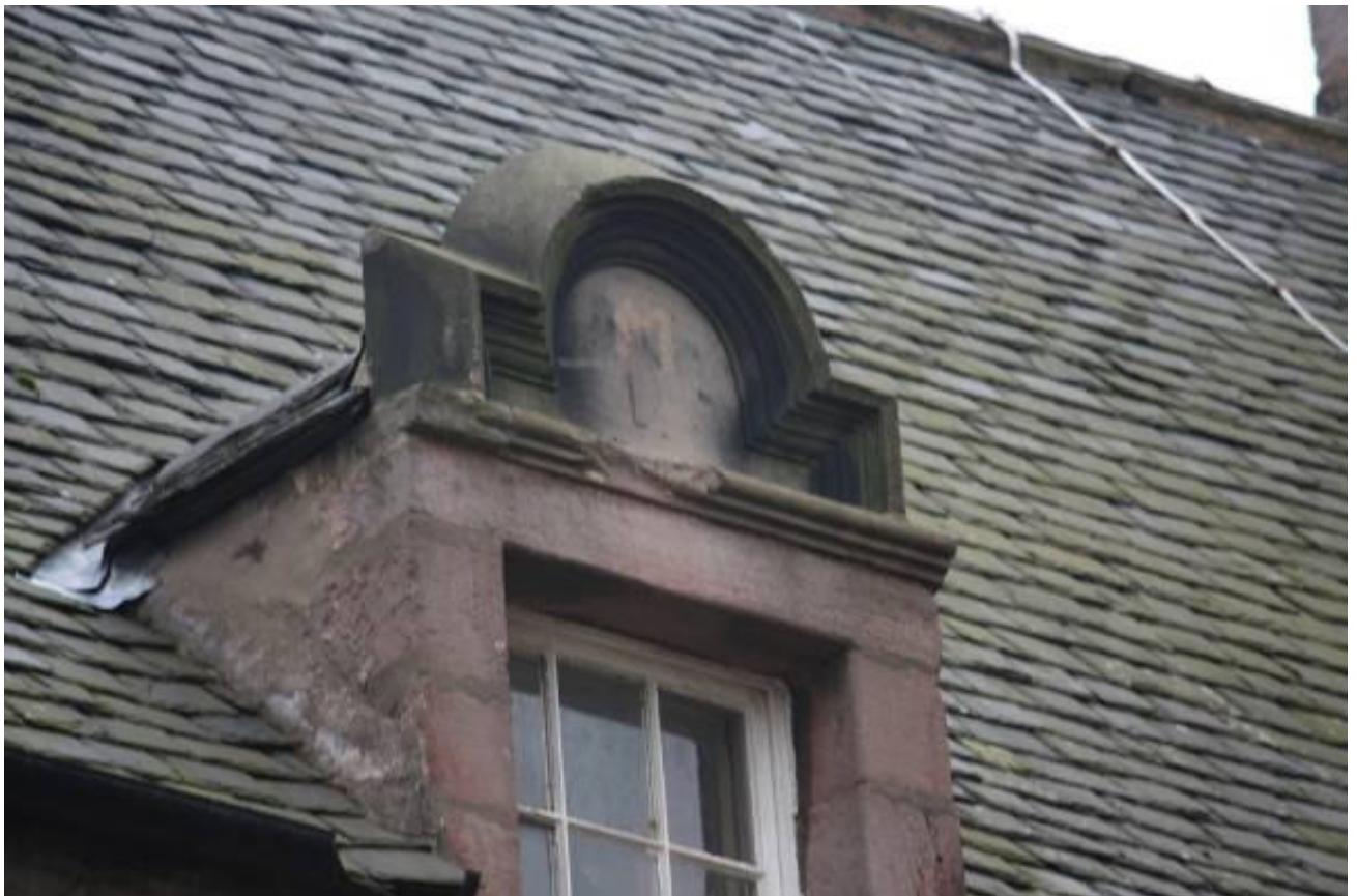
Lead flashing replaced with mortar around dormers
