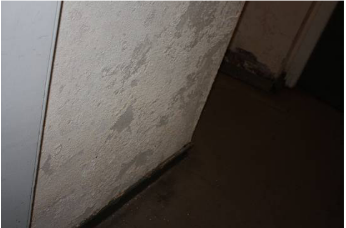
Evidence of damp internally at ground floor
