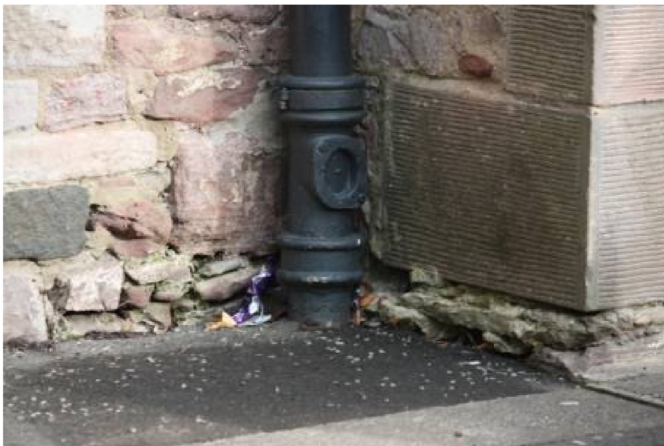
Evidence of damp and stone decay to base of Bruntsfield House – South elevation
