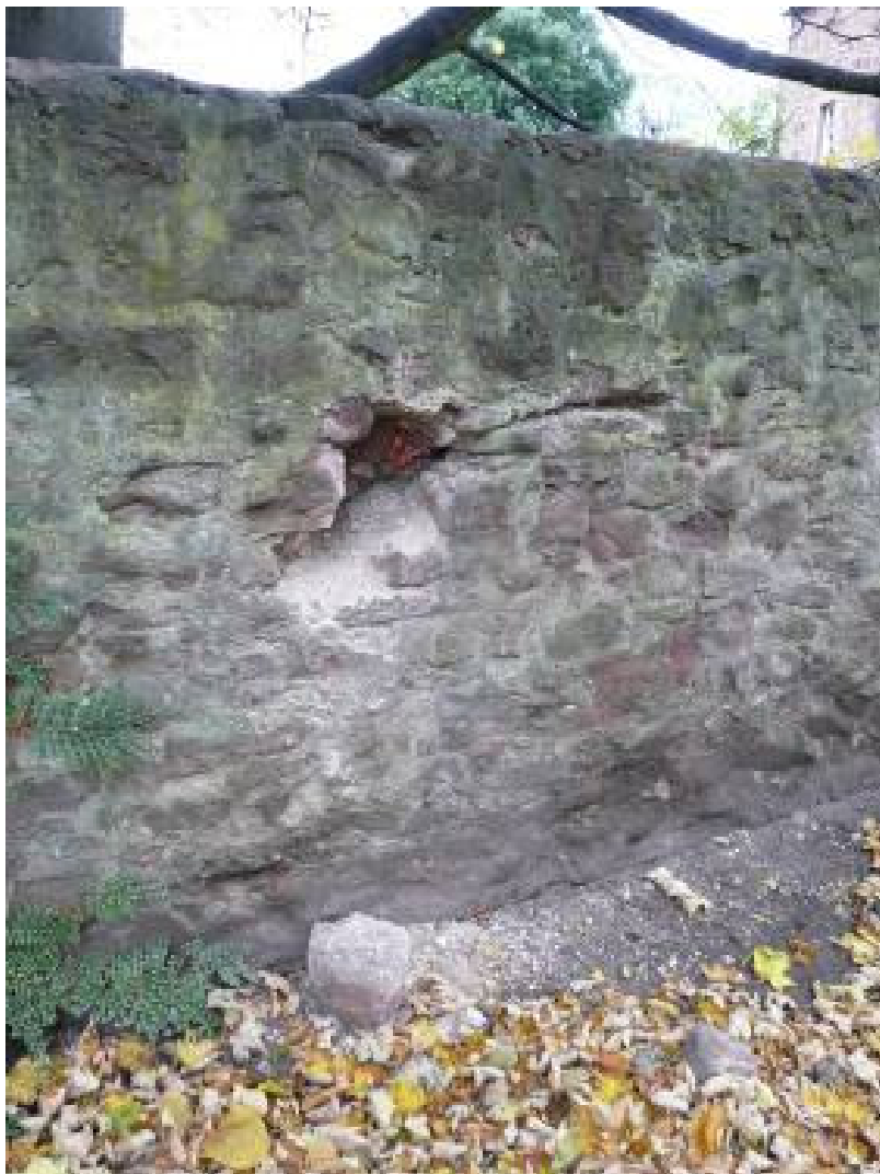
Missing stone and copes to driveway boundary
