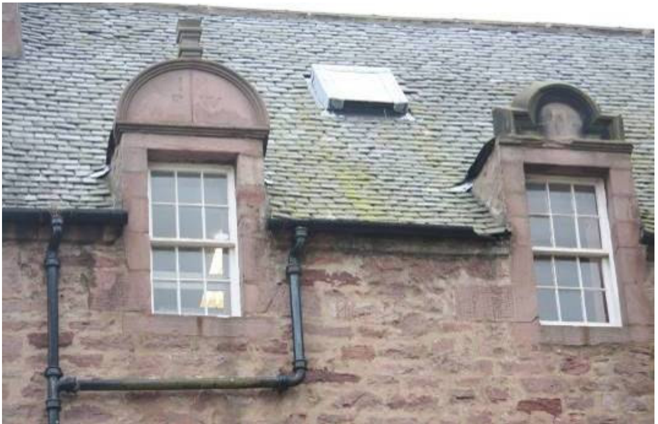
Staining to north elevation due to damaged rainwater goods
