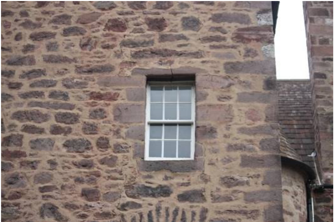
Crack to lintol above top floor window, south elevation
