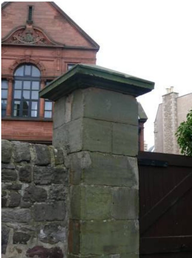
Damage to ashlar gate pier
