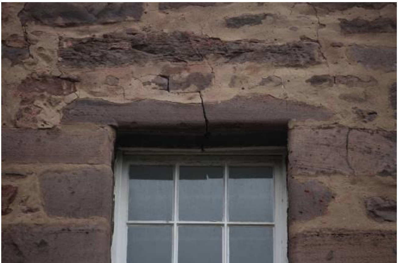
Crack to lintol above top floor window, south elevation
