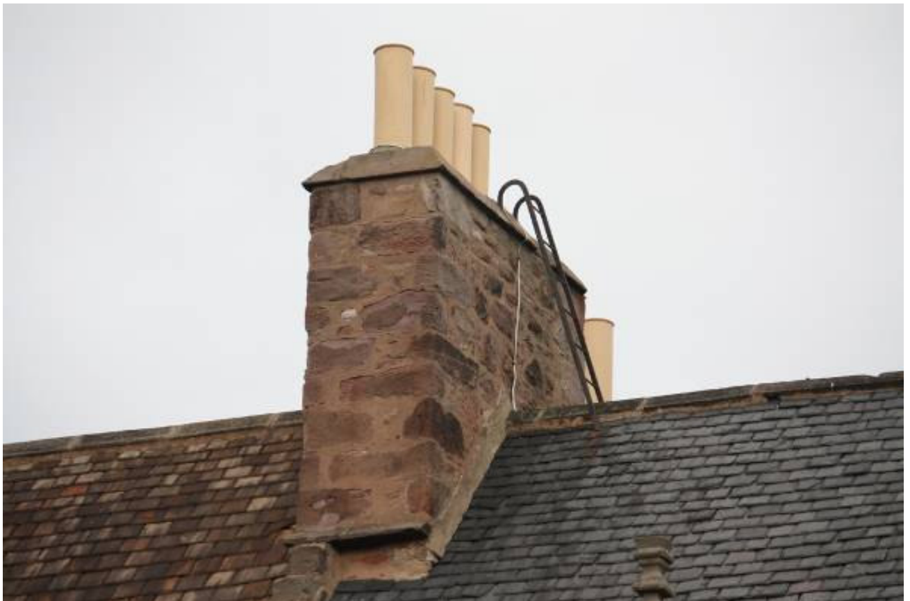
Deterioration to stonework on chimney and ridge of slate roof
