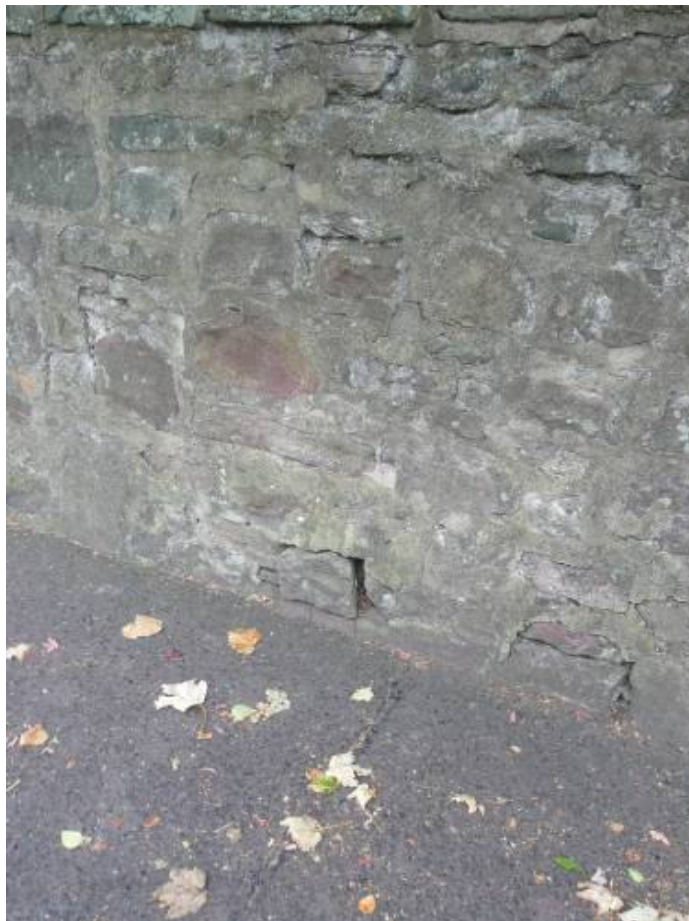
Dislodged and missing stones
