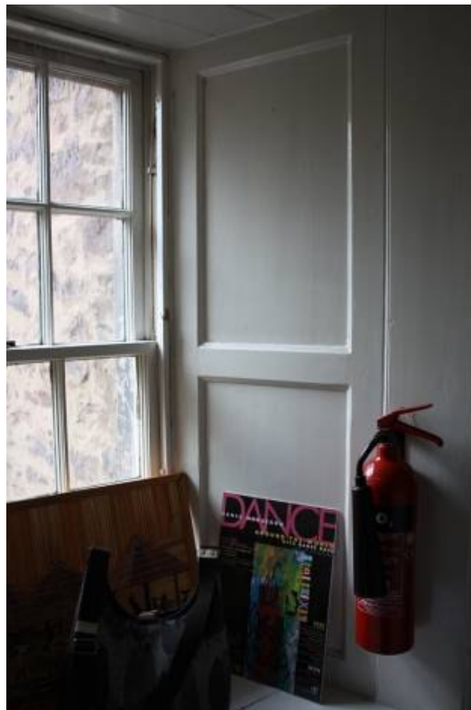
Example of window with mix of tongue & groove and raised and fielded panelling
