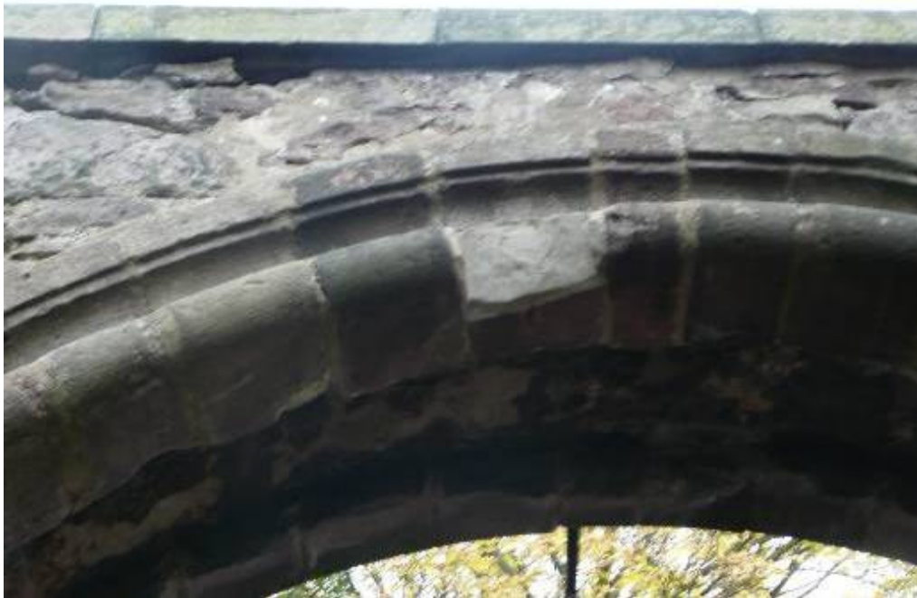
Damage to arch connecting to Bruntsfield House
