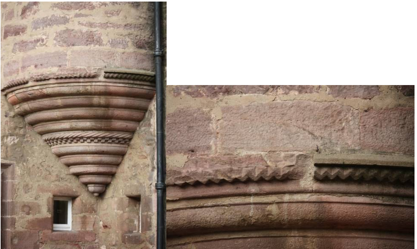
Missing carved stonework to base of stair tower turret
