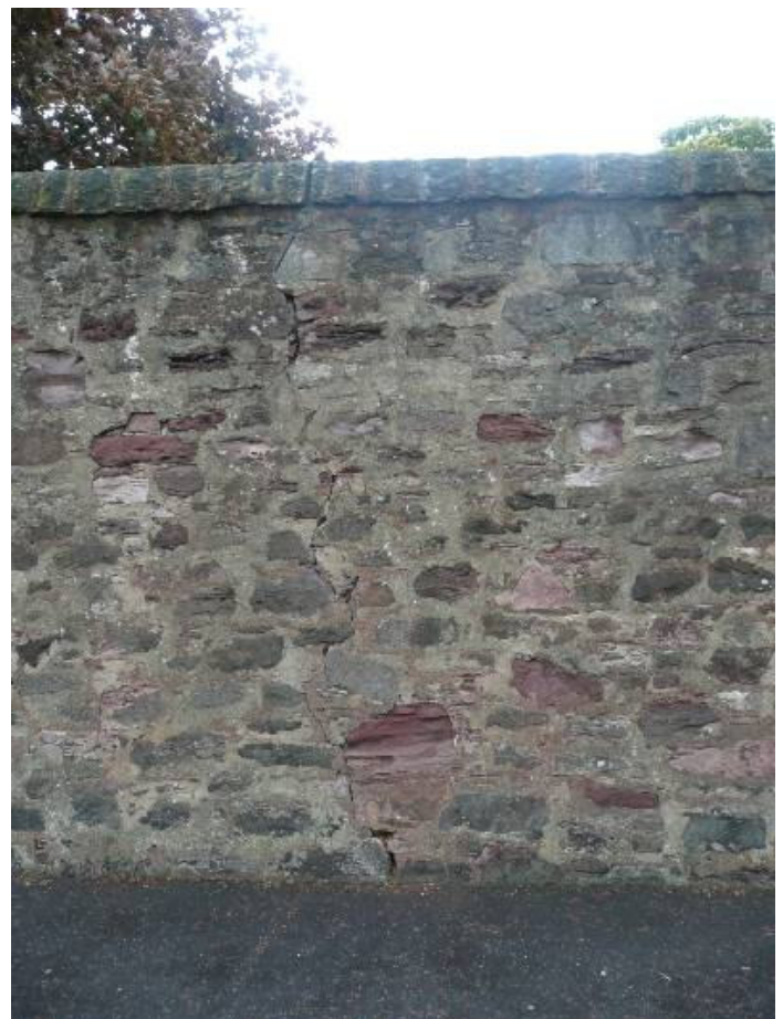
Cracks through wall
