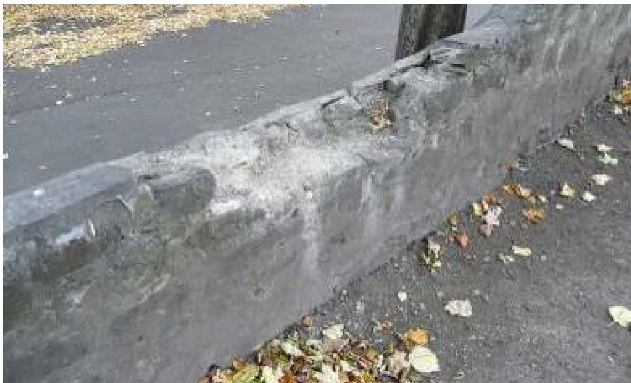
Missing stone and copes to driveway boundary
