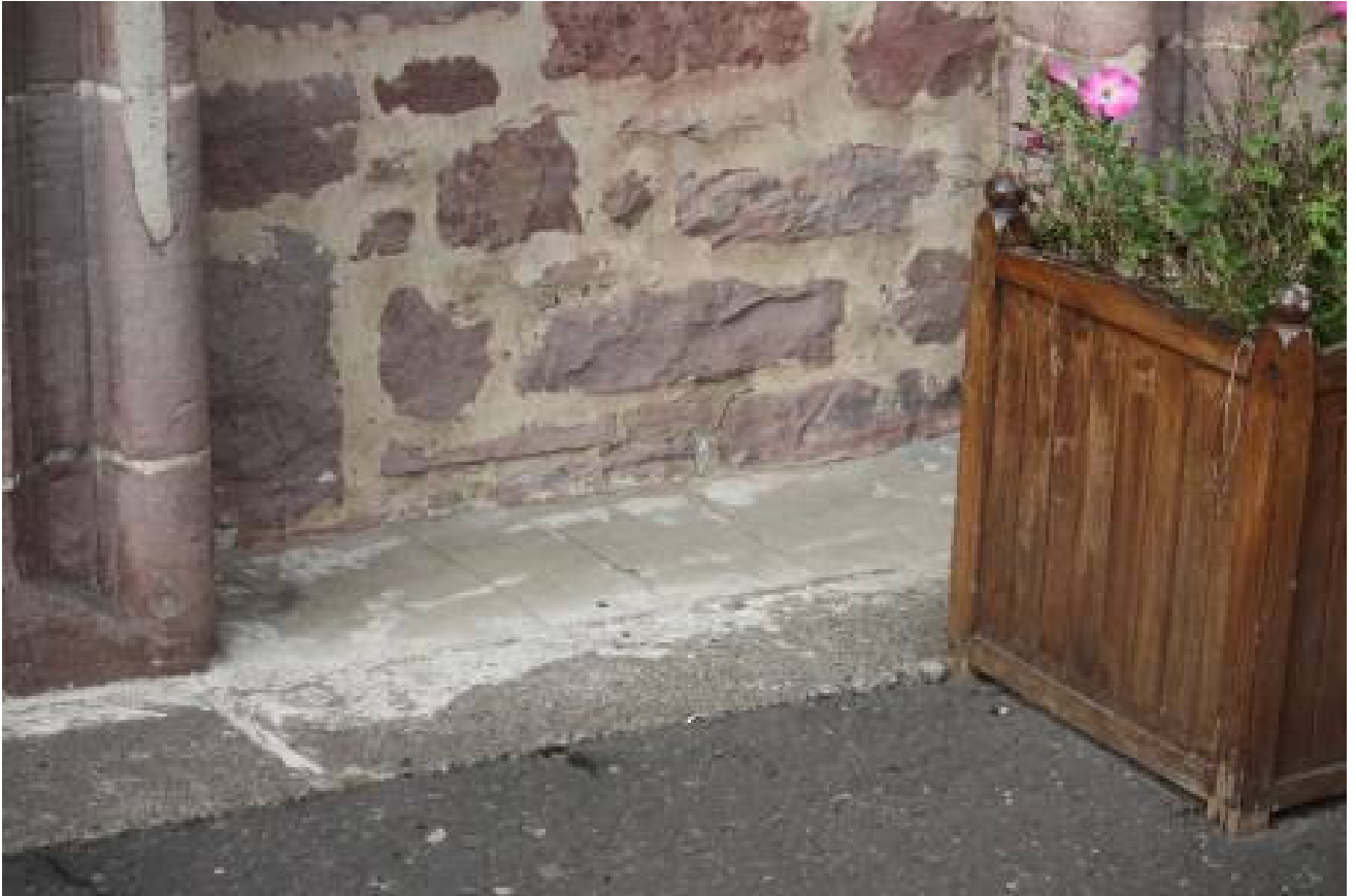
Mortar Seal on east elevation
