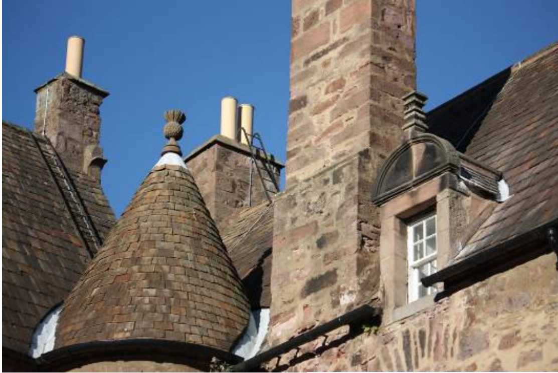
Decay to stonework at base of chimney
