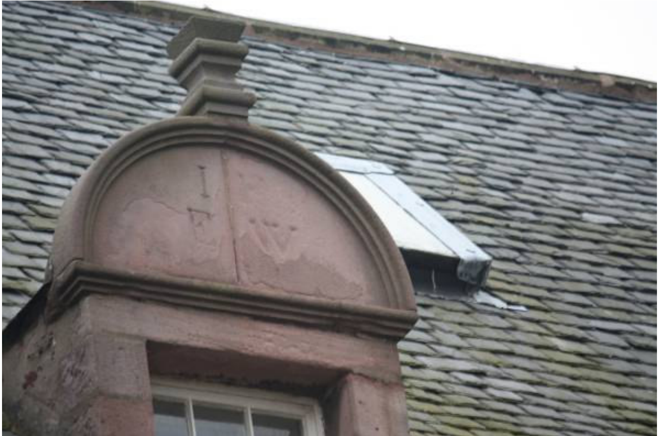
Delamination and wear to carving above window
