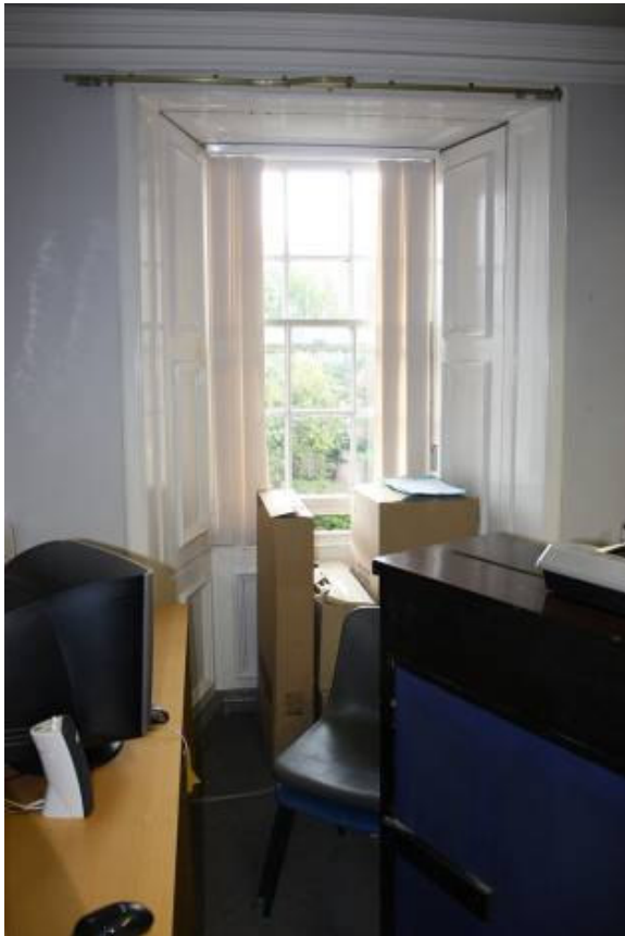
Typical panelling to ingoes with shutters
