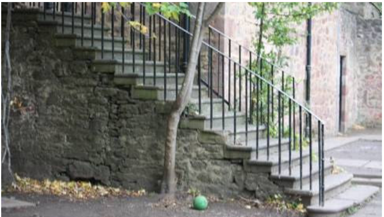
Staircase to Head Teacher's office showing damage to stone structure, steps and balustrades.
