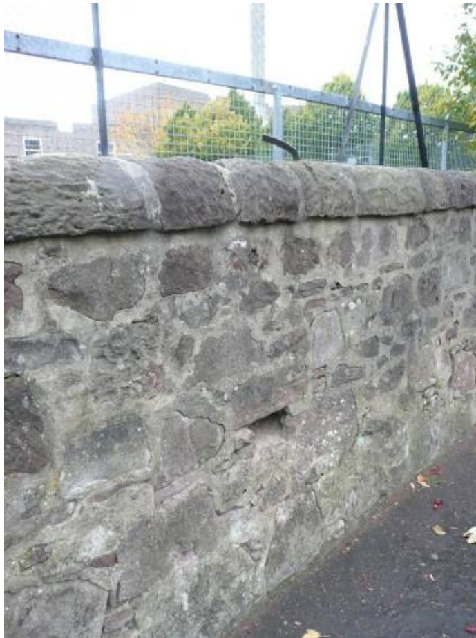
Dislodged and missing stones
