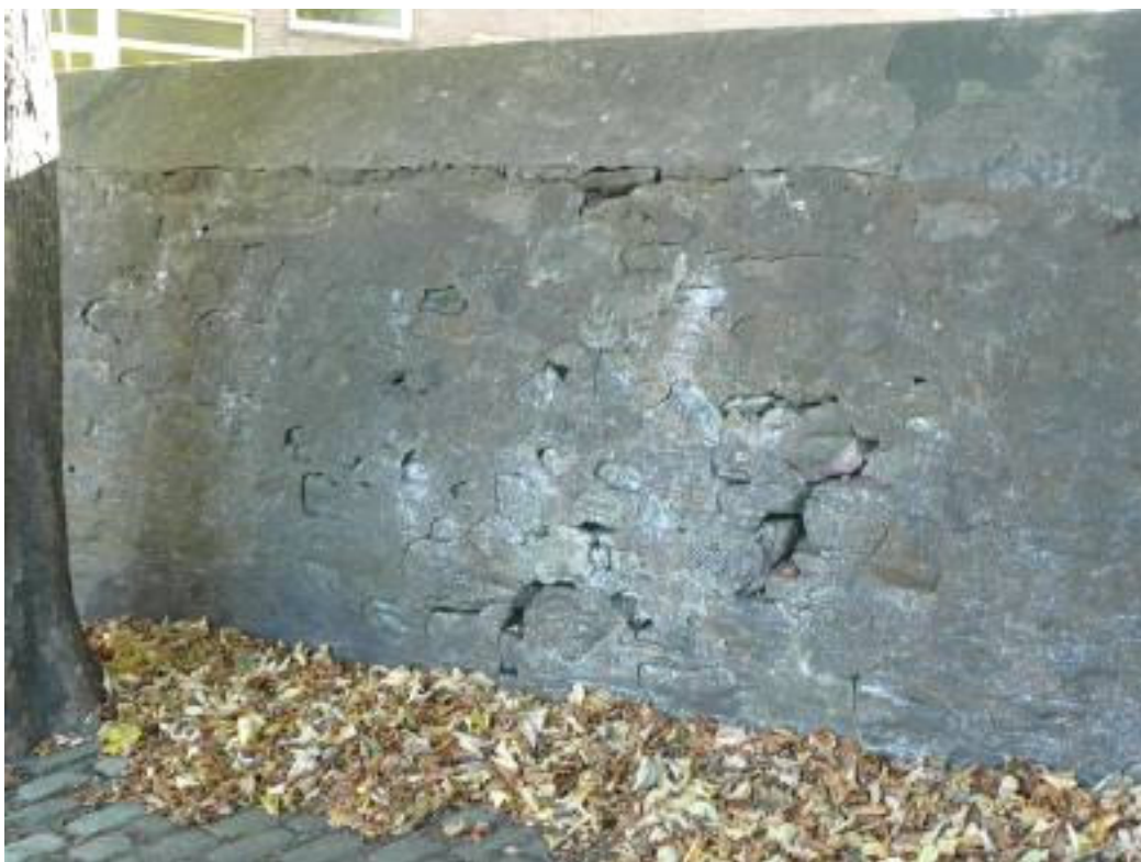
Area of stone affected by incorrect mortar
