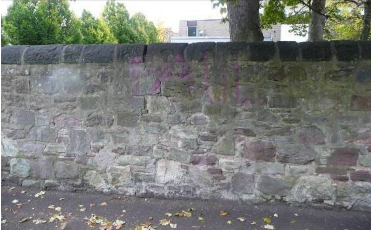
Damage to stonework and copes on north boundary wall
