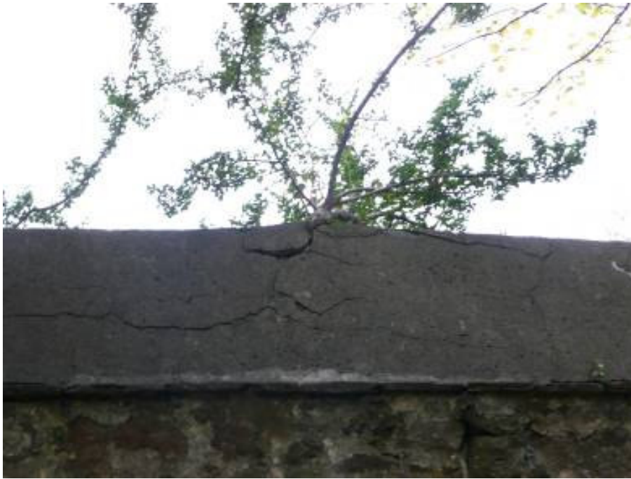
Plant growth affecting pyramidal mortar cope
